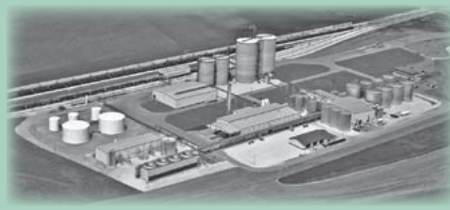
Fagen, Inc., 100 million gallon per year ethanol plant
